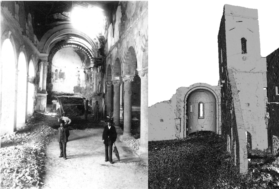
Fig. 7 – Comparison between the historical images of the interior of the Church (after 1895) and the 3D geometric model (Copyright: ArTeSalVa project)
