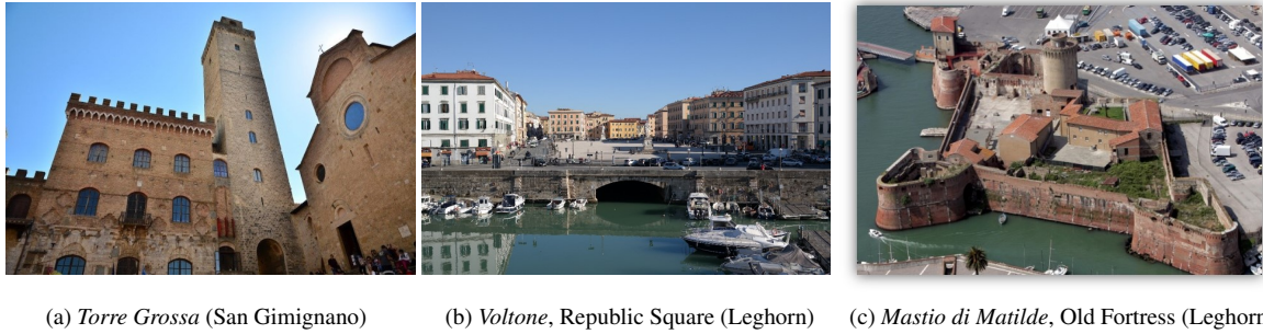
FIGURE 2: Three case studies under analysis in the MOSCARDO project; all sites are located in Tuscany, Italy. The Mastio di Matilde is the large round tower (in the top center) pertaining to the Old Fortress in Leghorn; the Voltone is the waterway below a large town square; the Torre Grossa is the tallest of the historical towers in the city of San Gimignano, close to Siena.
