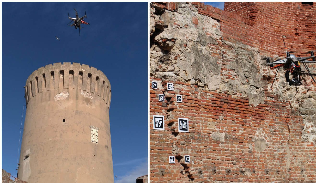
FIGURE 5. The two main different tasks of the UAV in the proposed IoT system: on the left, image acquisition for 3D reconstruction; on the right, periodical image acquisition for marker-based structural defects monitoring.
