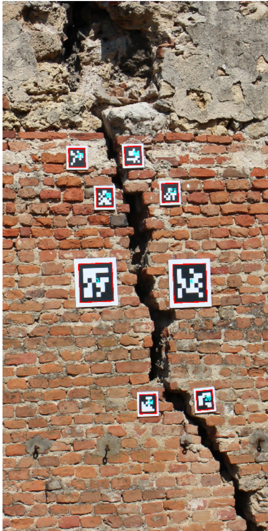
Figure 3: Four pairs of markers, correctly detected and identified.
