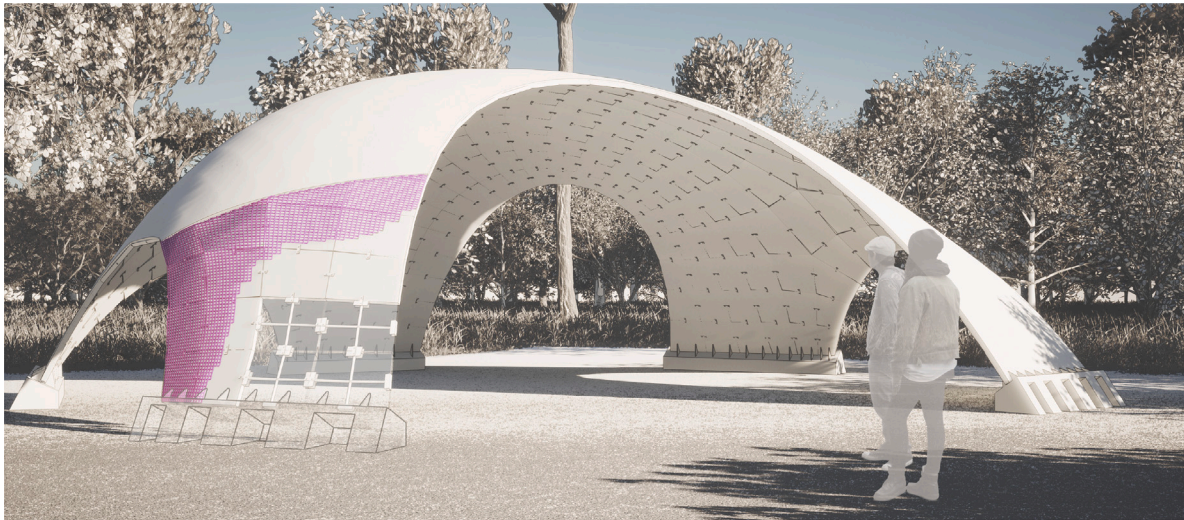
Fig. 1. Conceptual view with technical details of our concrete shell: the shape is segmented into flat tiles that are jointed at the midpoint of the edges and post-tensioned; the outer surface is finished with wire patches and in situ casting.
