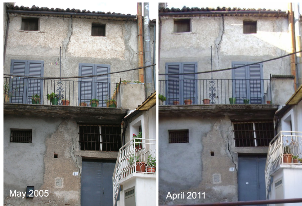
Fig. 4 Photo survey clearly indicating the increase in lesions, across the 2005–2011 period, affecting a building located in the historical centre
