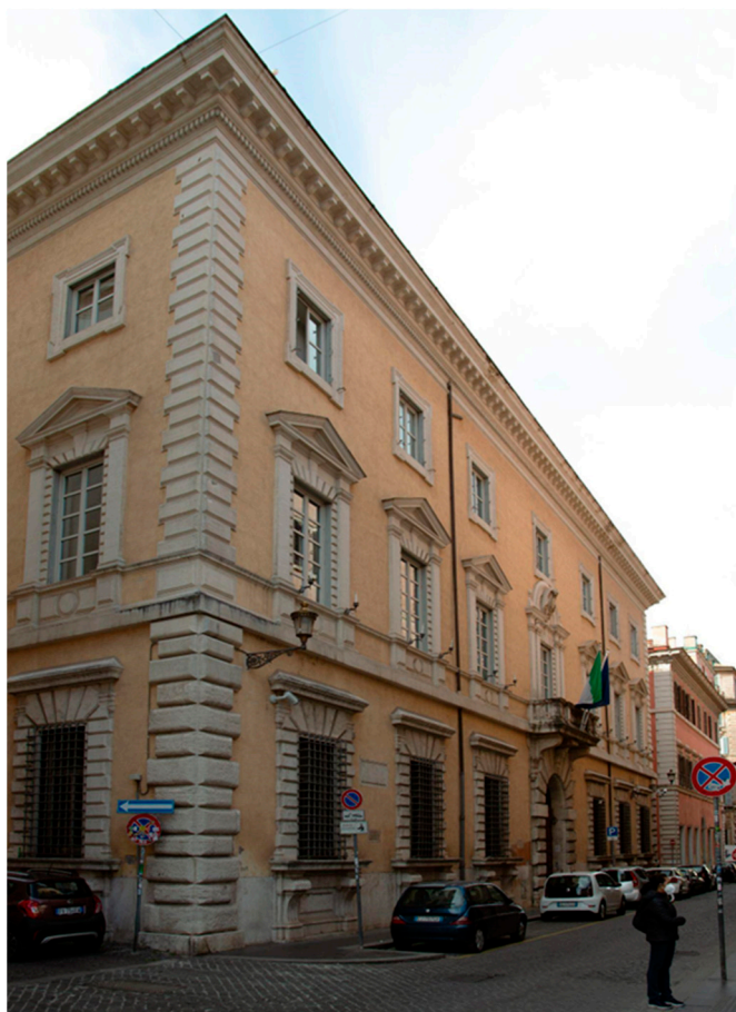
Figure 2. Palazzo Maffei-Borghese, Rome, Italy.
