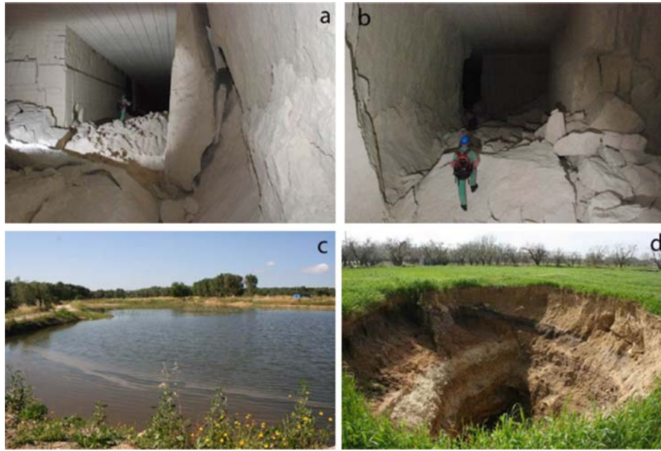
Figure 12. Instabilities in the underground quarries (a and b) and examples of sinkhole at Cutrofiano (c and d).
