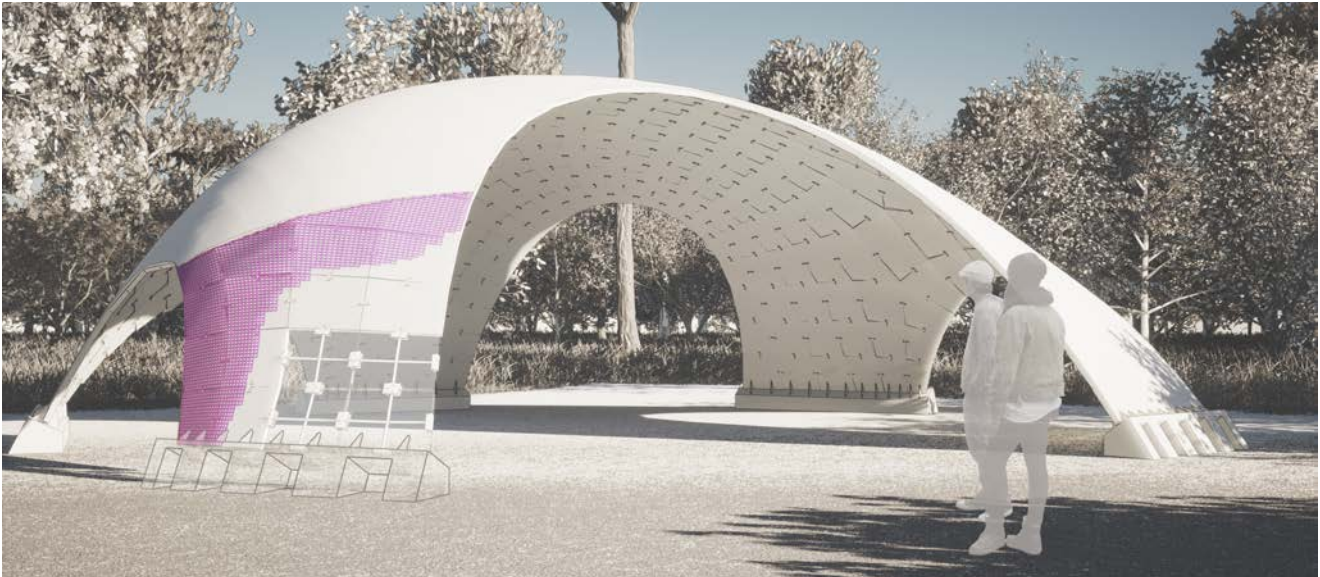
Figure 1: Conceptual view with technical details of our concrete shell: the shape is segmented into flat tiles that are jointed at the midpoint of the edges and post-tensioned; the outer surface is finished with wire patches and in situ casting.
