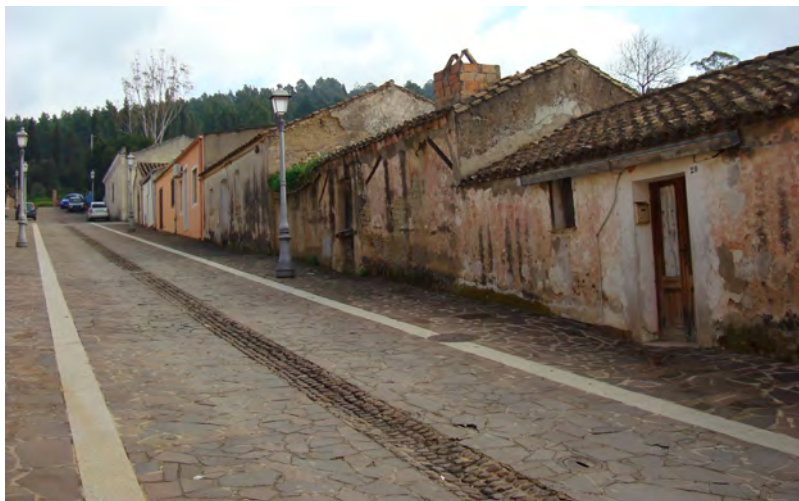
Fig. 3 Sa Domu 'e Pasci, Santadi (SU), exterior of building before restoration (Photo Paolo Paschi)
