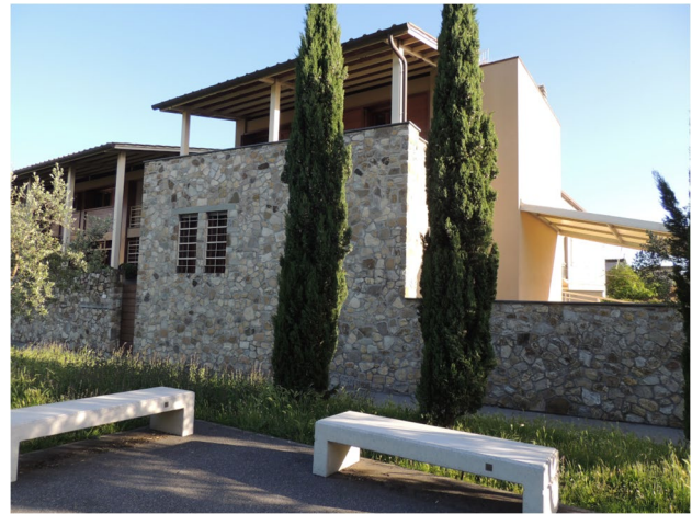
Fig. 30 Cladding of a decorative structure in Sesto Fiorentino (Florence)
