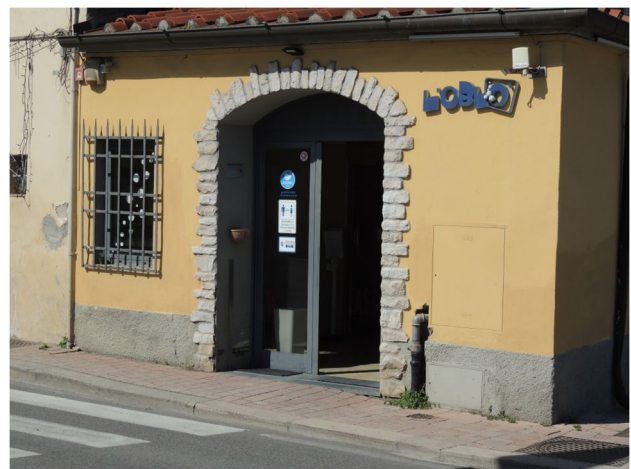
Fig. 29 Cladding in imitation of false bases in Calenzano (Florence)
