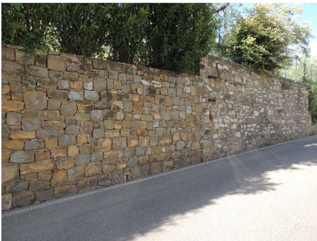
Fig. 33 Recent reconstruction of a boundary wall where a carbonate stone different from Pietra Alberese was used (Calenzano, Florence)
