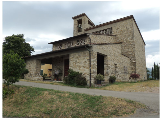
Fig. 27 The Church of Santi Pietro and Girolamo, in the hills south of Pistoia with roughly hewn ashlar of Pietra Alberese used together with Pietraforte sandstone
