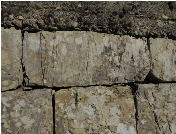
Fig. 9 Fracturing along calcite veins
