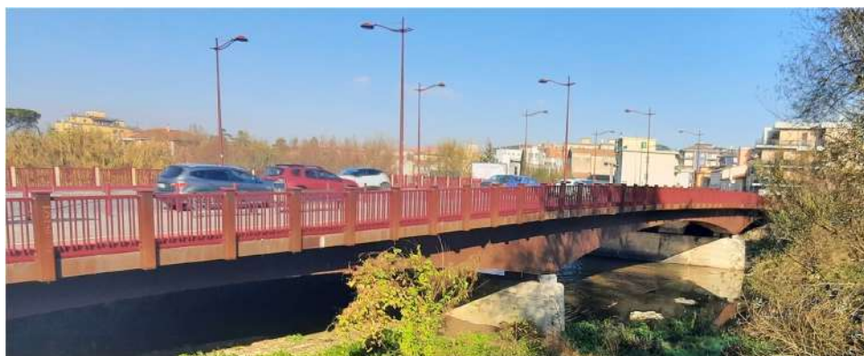
Figure 17. Santa Maria degli Angeli Bridge crossing the Sabato River today (photo by F.T. Gizzi).
