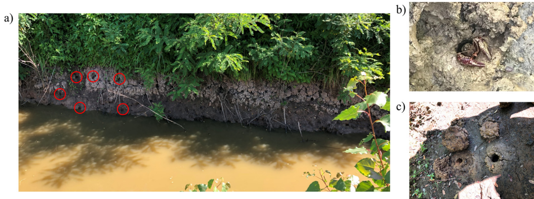
Fig. 2. Picture of a channel bank affected by burrowing activity: (a) highlights of the burrows entrances (red circles); (b) P. clarkii in the burrow; and (c) burrows with a plug covering their entrance to maintain soil moisture.
