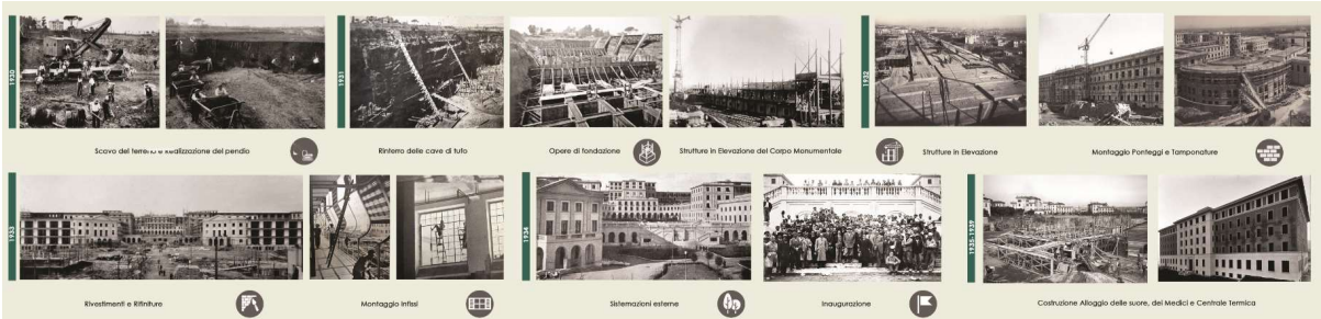
Fig 4: Construction steps of the hospital complex.
