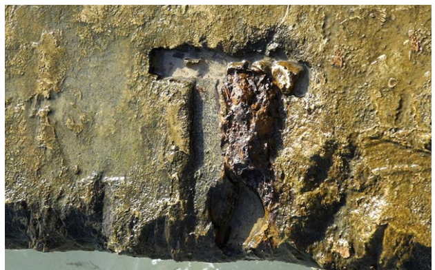
Figure 12: Example of “T” shaped next to “C” shaped clamp.
