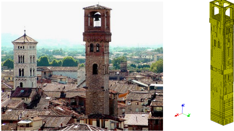
Fig. 2 The Clock Tower and the finite-element mesh.
