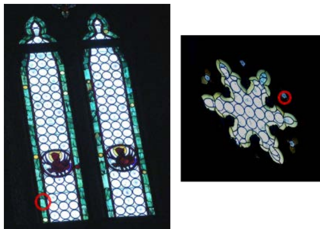
Figure 2. Windows of the Basilica di San Giovanni e Paolo from which the fragments were selected. The red circle shows the location from which the fragments originate (SSGP1 and SSGP2 left, SSGP3 right).
