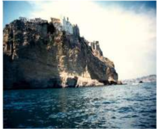
Figure 10. Detail of the Terra Murata coastal cliff, showing the stratigraphy of the pyroclastic successions having different technical characteristics.
