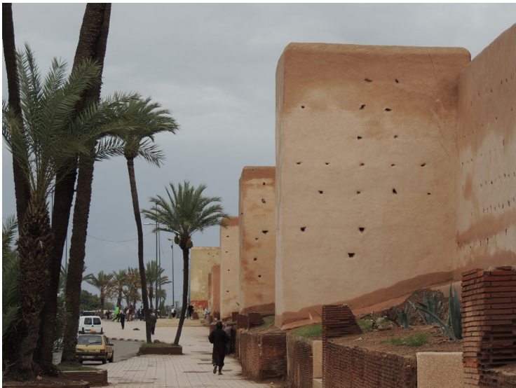
Fig. 11 The earthen plastered city walls of Marrakech
