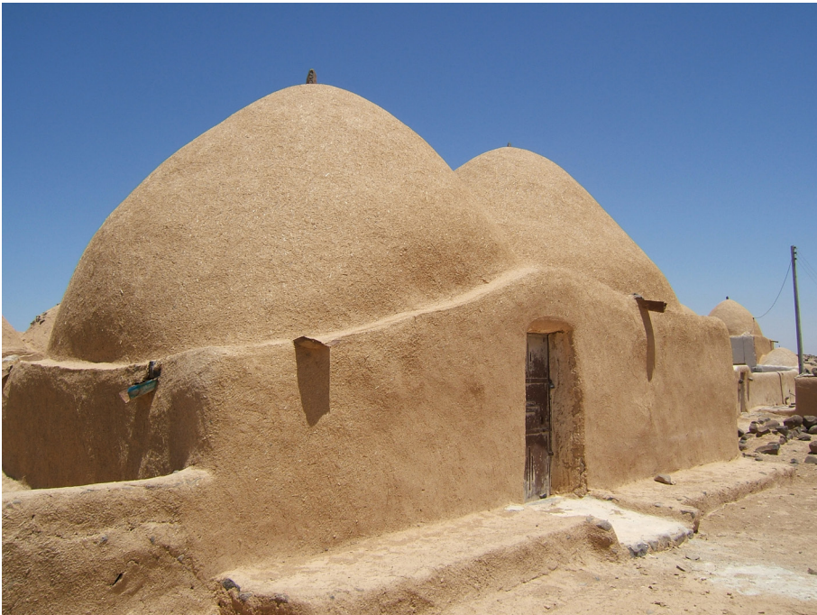
Fig. 2 Syrian corbelled dome house, well maintained
