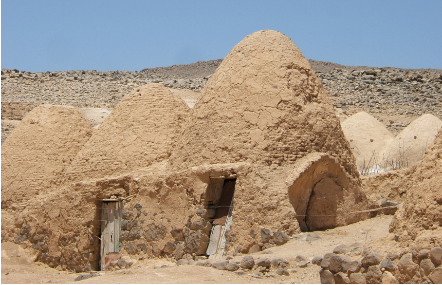
Fig. 3 Syrian corbelled dome house, lack of maintenance
