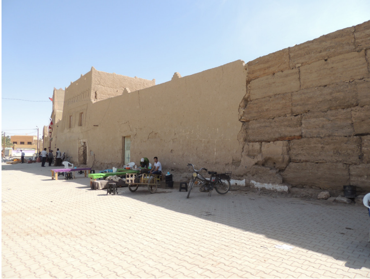
Fig. 10 Ongoing works to protect with an earthen plaster the walls of a village in Morocco
