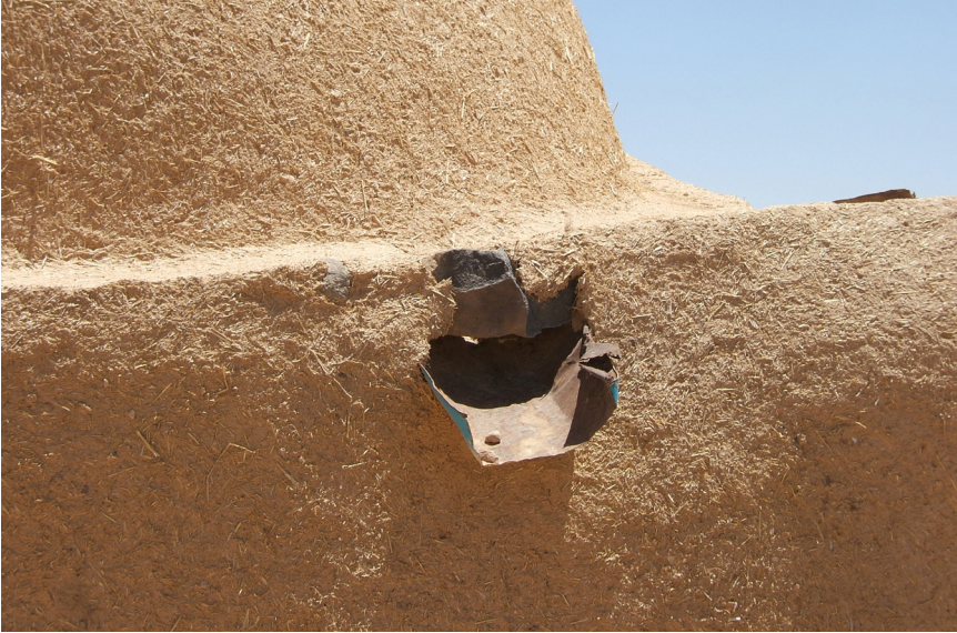
Fig. 8 Improvement of the water run-off to avoid concentrated flow on the walls in a Syrian corbelled dome house
