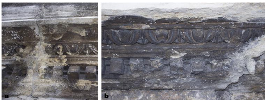
Fig. 1. Details of the decorated sub-frame of Palazzo Verità Montanari in Verona (fotos from 2016) with (a) calcium carbonate recrystallization phenomena and (b) black dendritic crusts (Lucrezia Campana, credits)
