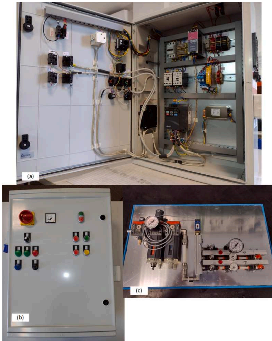
Fig. 23. Picture of the Internal View of the Electrical Cabinet (a), External Front View (b) and the Pneumatic Panel (c).
