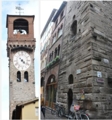
Figure 1. The Clock Tower in Lucca: upper part and ground floor
