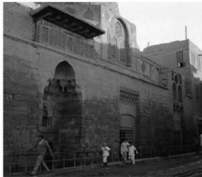
Fig. 21. EXTERIOR OF THE MAUSOLEUM BEFORE AND AFTER RESTORATION
