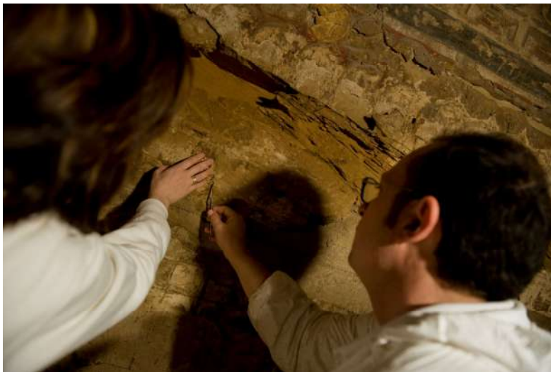
Fig.19 - Room XII, consolidation of the rock - photo by ARCE
