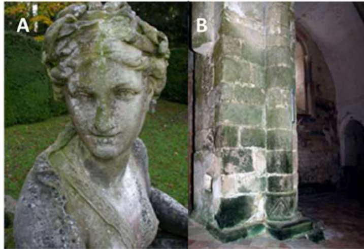
Fig. 1 – Algae colonization on a sculpture (Courances castle park) (A) and on a pillar (Les Salles-Lavauguyon church) (B) 49 .
