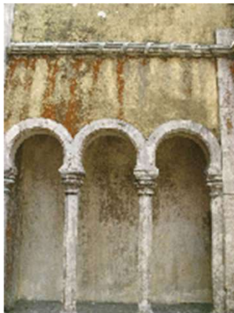
Fig. 2 – Discoloration phenomena on Palácio Nacional da Pena (Portugal) colonized by Trentepohlia , Cyanobacteria 50 .
