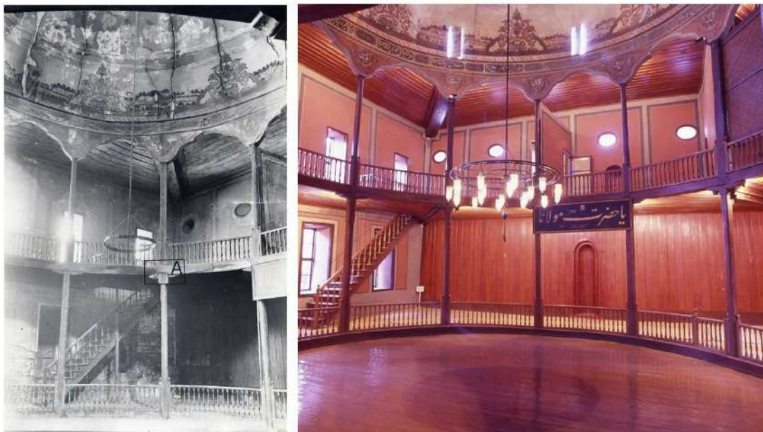
Fig. 4. INTERIOR VIEW OF THE SAMAKHANA BEFORE AND AFTER RESTORATION
