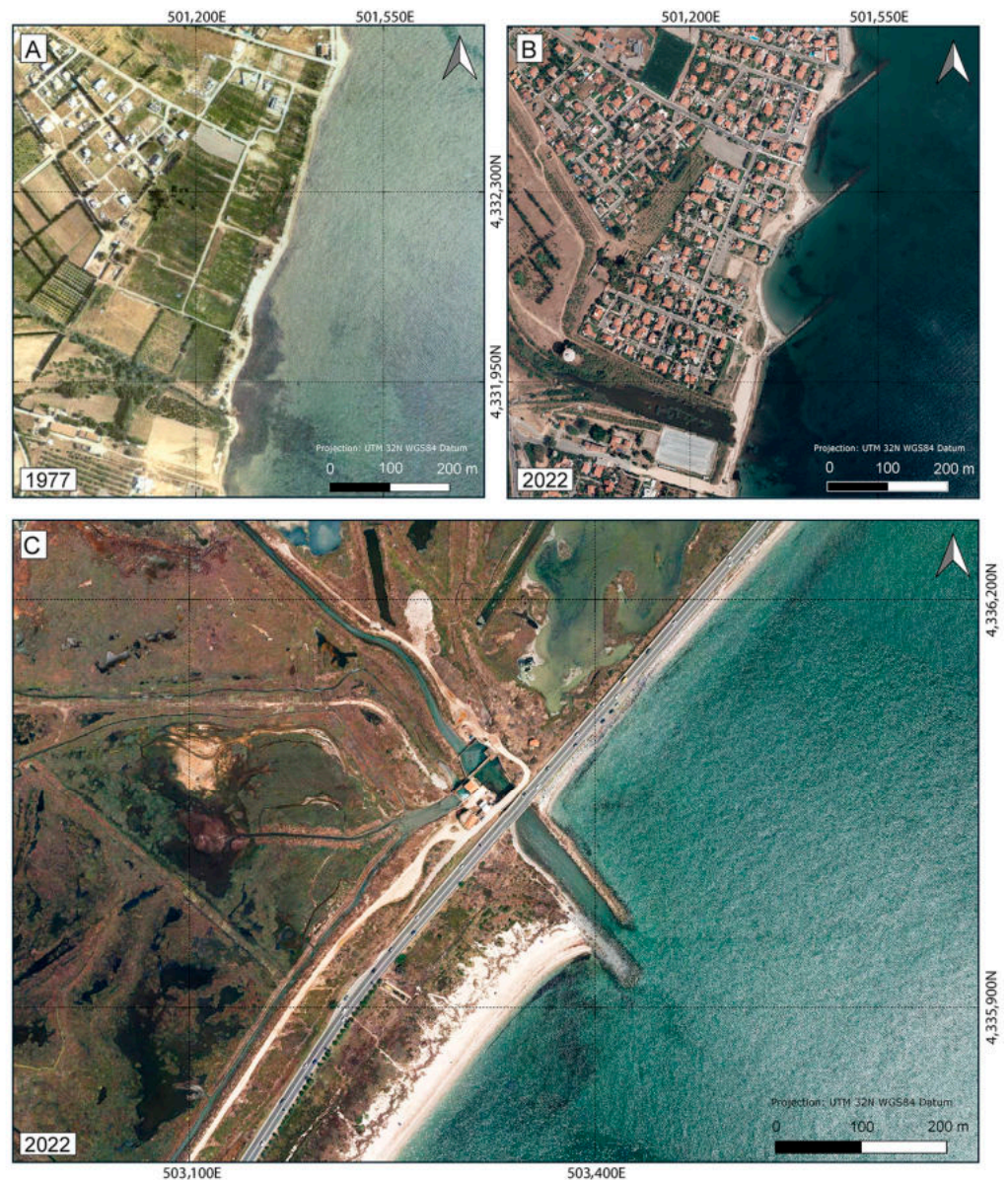
Figure 12. Panels (A,B) show beaches ID 43 and 44 (Frutti d’Oro Beach), which are bordered by oblique groynes that have caused severe retreat. Panel (C) shows how the construction of two jetties across beaches ID 50 and 51 has interrupted longshore sediment transport, creating significant accretion in the updrift zone and significant retreat in the downdrift zone. Coordinate system: UTM 32N; Datum: WGS84.
