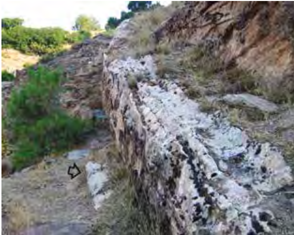
Fig. 66 North-eastern aqueduct in the hills east of Marmar Tepe: channel completely filled with calcareous deposits aligned with terracotta pipes (pointed by the arrow).
