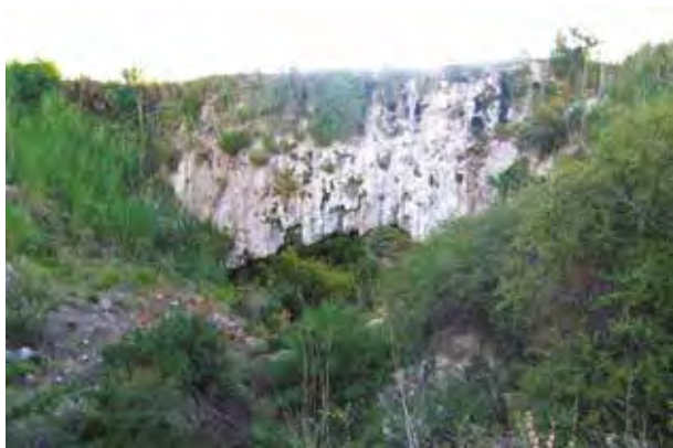
Fig. 75 The remains of the bridge used by a travertine channel in order to cross the Gök Dere.
