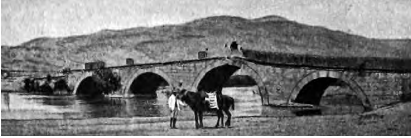
Fig. 88 The bridge of Ahmetli in a photograph taken in the late 19 th century, when the original ancient structure was still completely conserved (after Sarre 1896, fig. 1).
