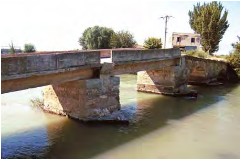
Fig. 91 The bridge of Ahmetli: the upriver side with the triangular cutwaters built to reinforce the piers.
