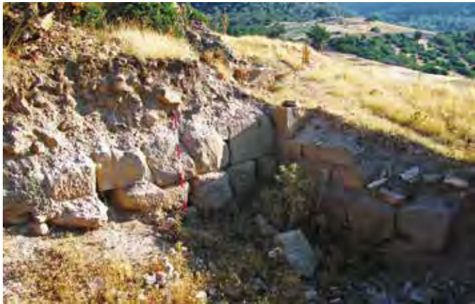
Fig. 24 Alaburun: structures at the south- eastern base of the tumulus.
