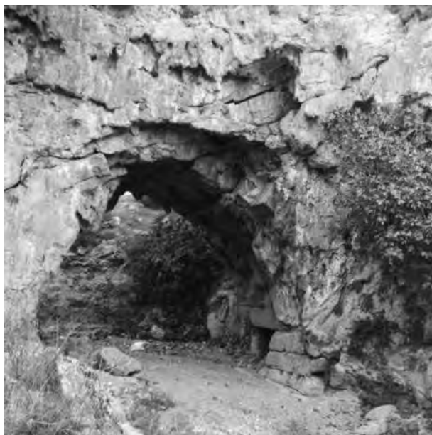
Fig. 73 The remains of the bridge on the Kadi Dere along the road between Hierapolis and Laodikeia, visible in a 1960 photo and now completely covered in calcareous deposits.
