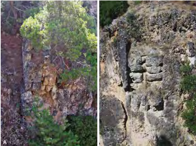
Fig. 62 North-eastern aqueduct: southern (A) and northern (B) abutments of a bridge on the course of the Gök Dere.
