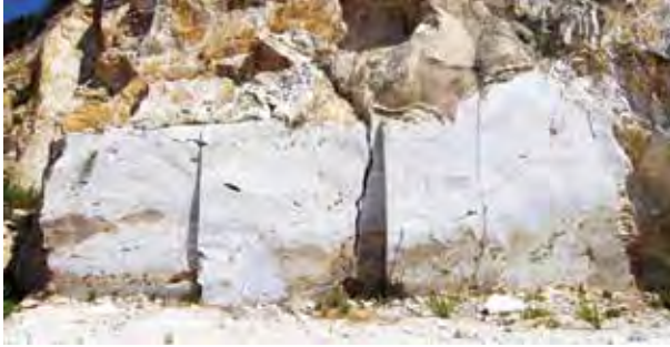
Fig. 138 The alabaster quarries of Gölemezli: modern quarry face (documented in 2006).
