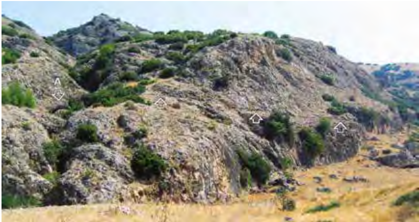
Fig. 57 Northern aqueduct: groove excavated in the rock to seat the terracotta pipes (see fig. 58), visible on the slopes east of Yokuşyol; an arch made of travertine voussoirs (A) is also indicated (see fig. 59).
