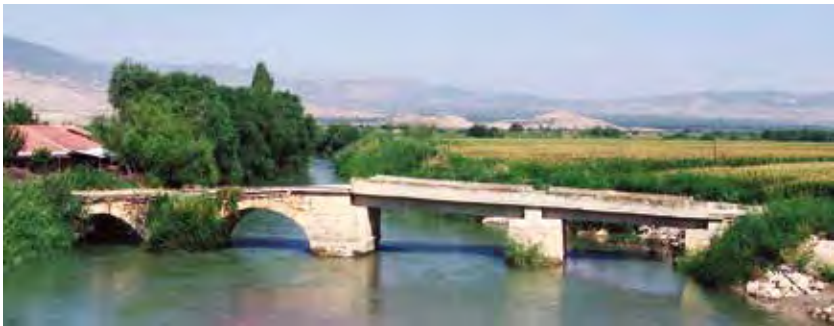
Fig. 89 The bridge of Ahmetli: general view from the south.
