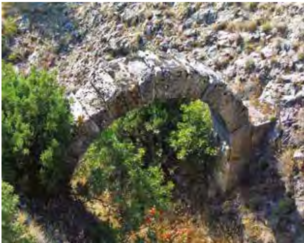
Fig. 59 Northern aqueduct: arch composed of travertine voussoirs in the Yokuşyol district allowing the pipe to bridge the narrow gorge created by a seasonal watercourse.
