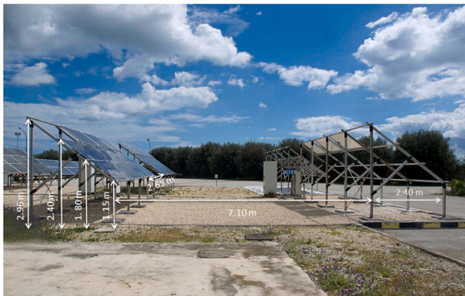
Fig. 3. Solar field with PV panels. Actual distances and heights are transferred in a simulation software.
