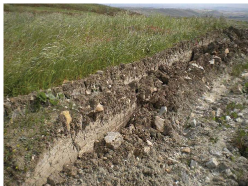
Figure 2. Typical slickensided shear surfaces along a continuous levee bounding the moving mass in a mudslide.
