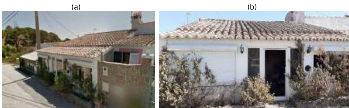
Figure 25 – General view of the building related to the “Faz Fato 1” episode: a) before the fire event (Google Earth image) and b) after the fire event (photo courtesy of Tavira Câmara Municipal).
