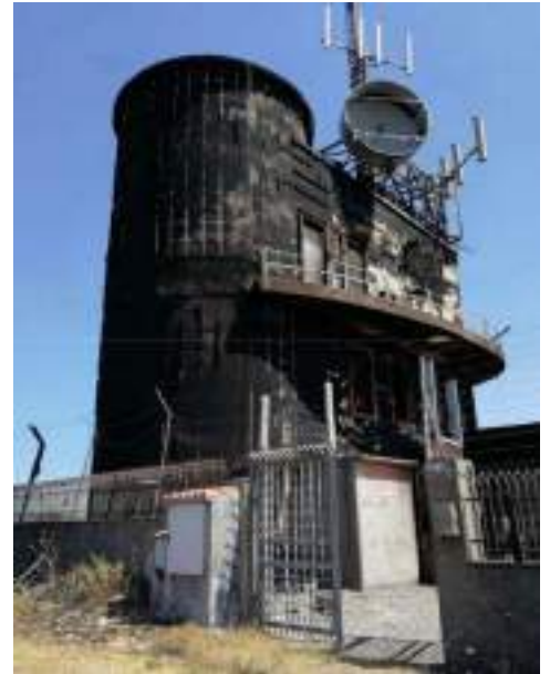
Figure 63 – Damage to a telecommunication infrastructure installed within a forest area affected by the fire (Source Protezione Civile).
