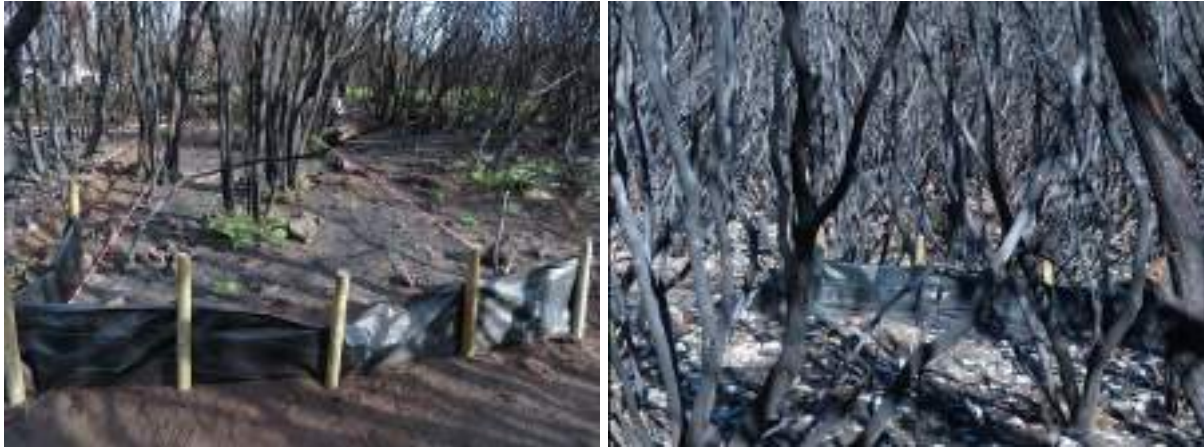
Figure 68 – The sediment fences installed in the Montiferru area a few weeks after the fire, prior to rain events.
