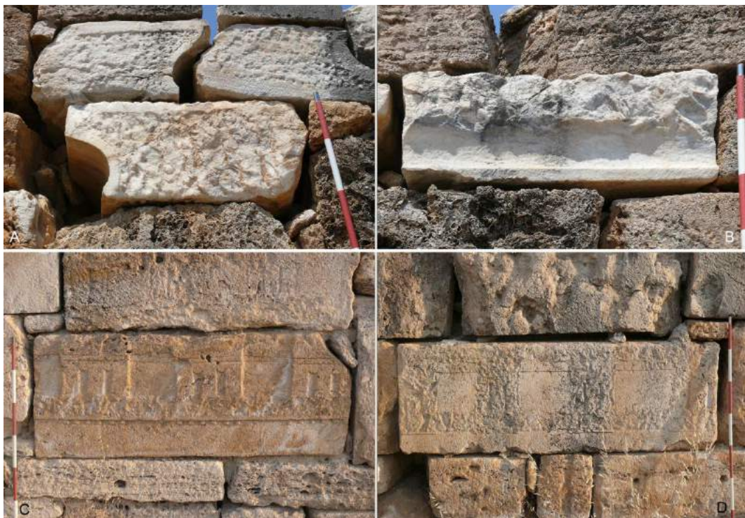
FIG. 12 – Example of blocks positioned in the outer curtain and deprived of the protruding mouldings (A-B: marble seats of the North Theatre; C-D: travertine frieze-architraves of the plateia ).
