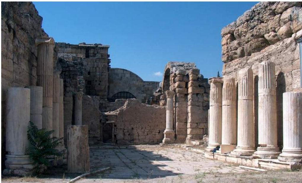
FIG. 23 – Great Baths, Hall H refurbished with Ionic columns taken from Temple B of the Sanctuary of Apollo.
