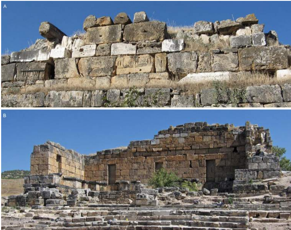
FIG. 22 – Nymphaeum of the Apollo Sanctuary: view of the main façade (B) and detail of the upper part of the rear wall reconstructed with spolia (A).
