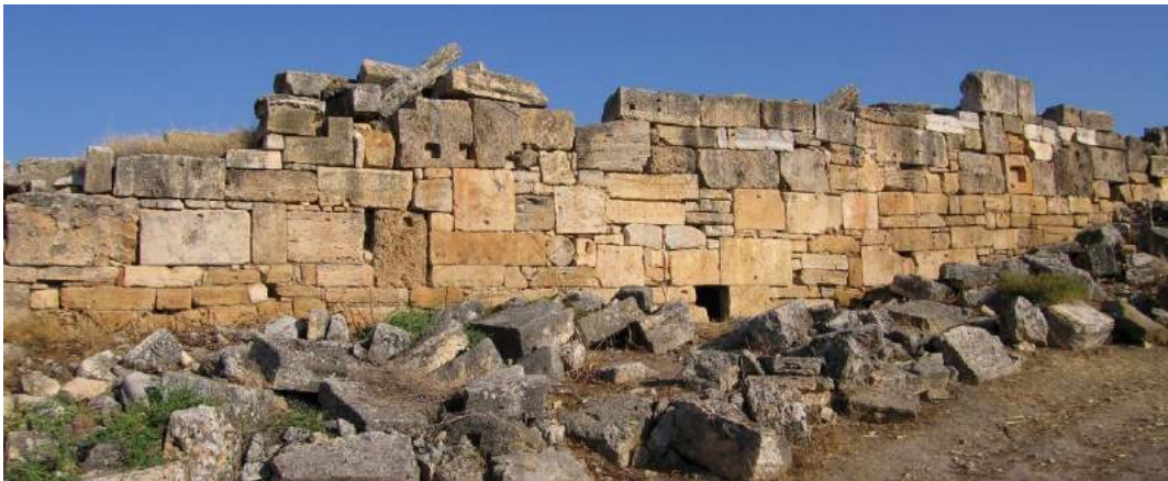
FIG. 3 – Stretch N of the city walls characterised by courses of blocks of different height, built on sloping terrain (Archive of the Italian Archaeological Mission).
