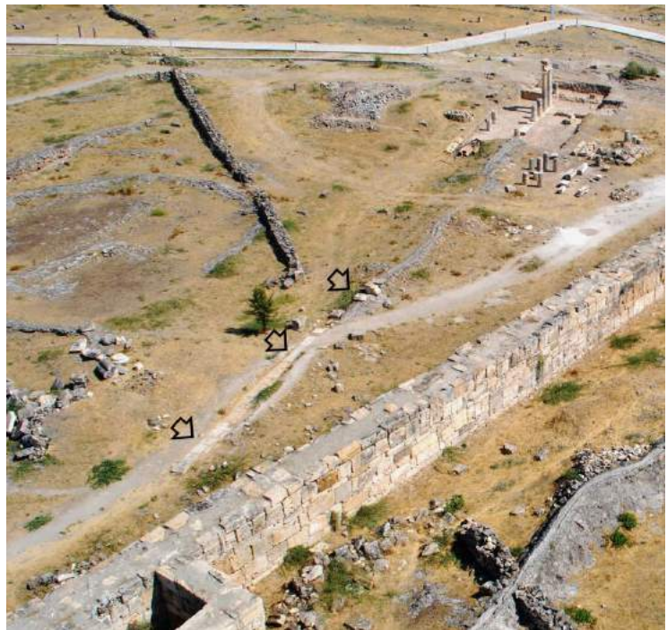
FIG. 20 – Gymnasium, aerial view of the stylobate of the south portico: the western sector was demolished during the construction of the city walls.
