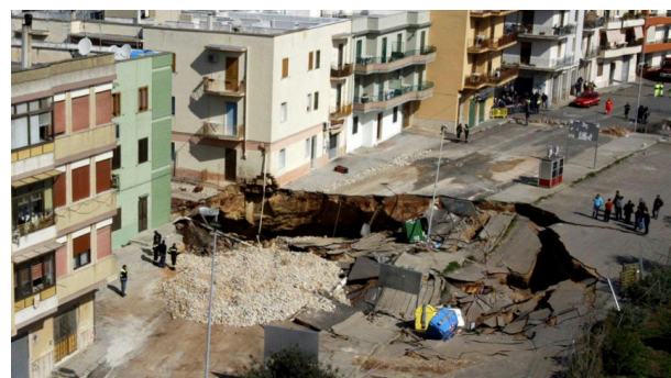
Figure 8. The March 29, 2007 sinkhole at Gallipoli (Apulia), a recent example of anthropogenic event due to an ancient underground quarry.
