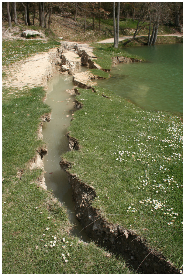
Figure 1. Development of cracks along the shores of Sinizzo Lake (Abruzzo), in the aftermath of the Mw 6.3 L'Aquila earthquake, on April, 6, 2009.
