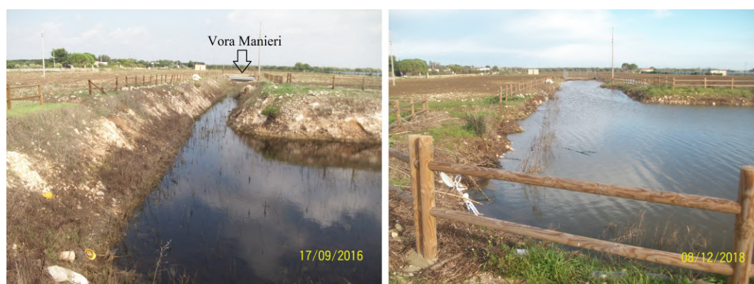
Figure 3. Hydrometric level of the final course of the new channel of the Asso Torrent; left: low after the first rains of the beginning of the 2016 wet season; right: high at the onset of a flood, resulting from moderate precipitation before 8 December 2018.
