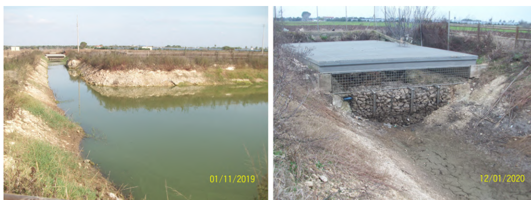
Figure 8. Left: the final course of the new channel in the beginning of November 2019; the hydrometric level was at a mean height, despite only 115 mm of rain in the previous four months; right: the entrance of Vora Manieri hole in the middle of January 2020; the brownish mud that covers the channel bed could cause clogging processes in the swallow hole.
