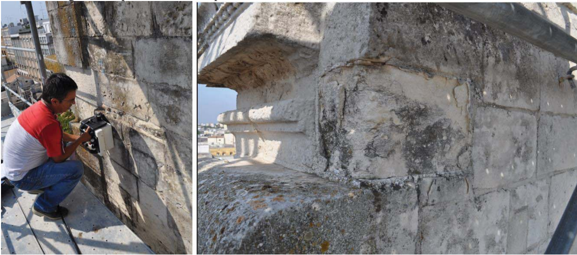
Fig. 2. Phase of the GPR data acquisition. On the right side of the photo, a detail of the status of conservation
