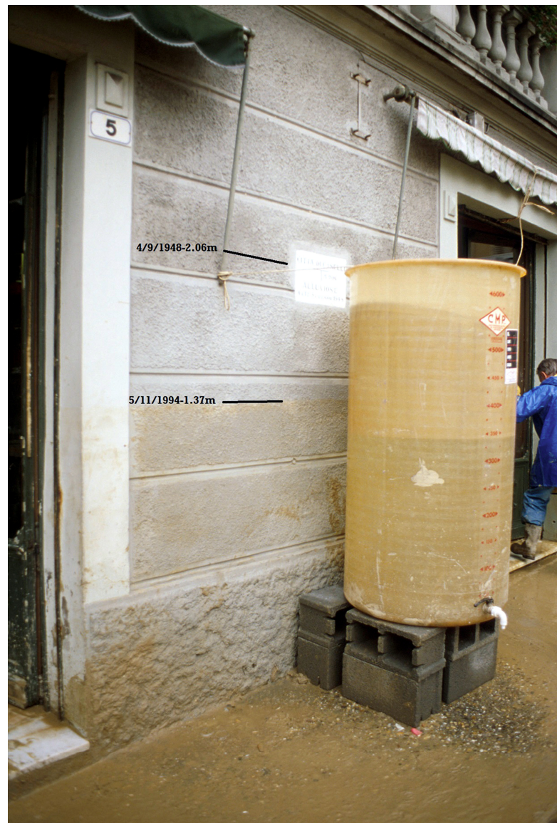
Figure 6. Canelli: In Cavour Square, marble marker of famous flood of 4 September 1948 compared with water level (meters) on 5 November 1994 (photo by F. Luino).
