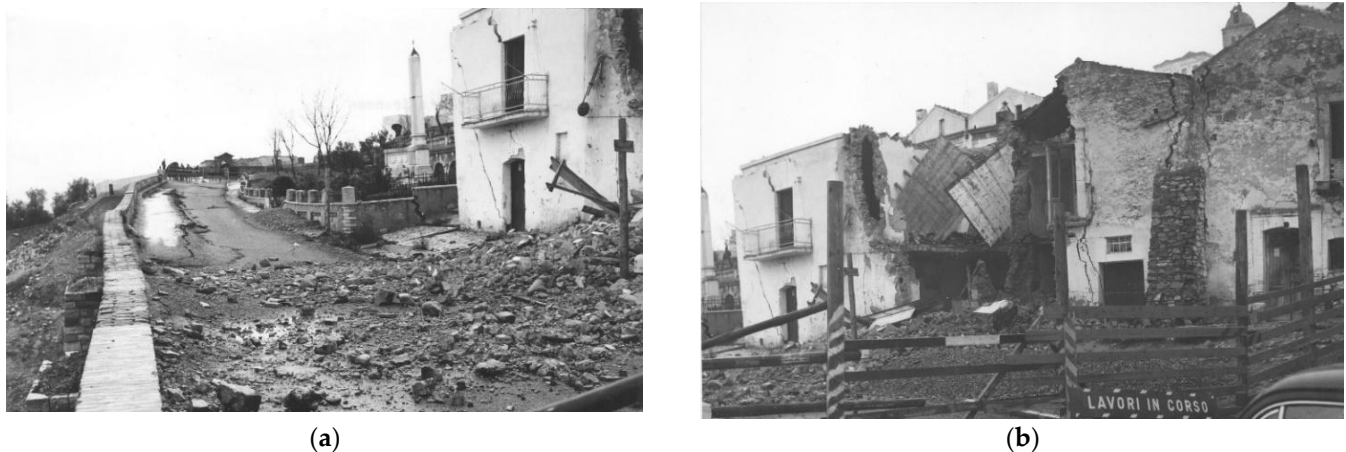
Figure 9. Effects of CS landslide reactivation in Craco in January 1965. (a) Area close to the retaining wall, damaged and partially collapsed due to landslide movement; (b) same areas with damage to residential buildings in foreground. A counterfort sustaining a building can be seen, indirectly suggesting old movements of the landslide [162].
