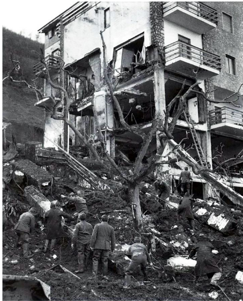
Figure 11. La Selva Hotel partially destroyed by mudslide of 2 January 1971 [72].
