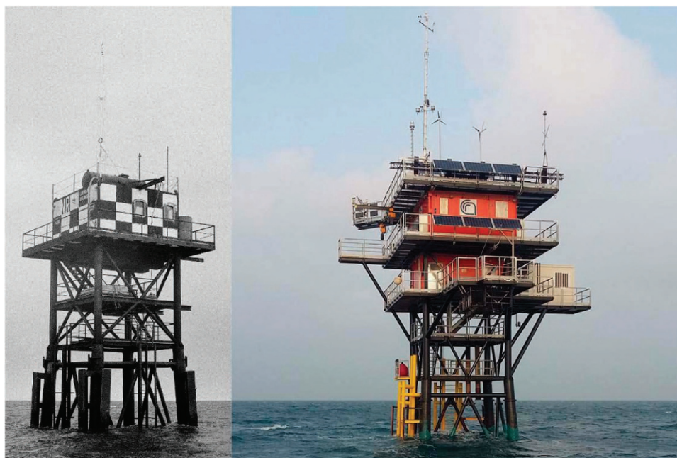
Figure 2. The Acqua Alta oceanographic tower. (a) In 1970, soon after its positioning, and (b) in 2017.
