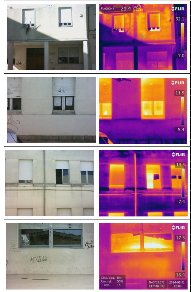
Fig. 4. Preliminary evaluation of thermal bridge for identify the ideal location for the placement of HFM instrumentation.
