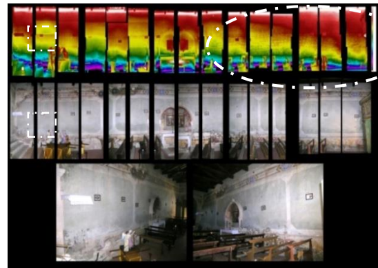
Fig. 7. S.S. Annunziata Church: Thermogram (top) and photograph (bottom) captured on June 15 th , 2007 inherent to the right wall from the inside part
