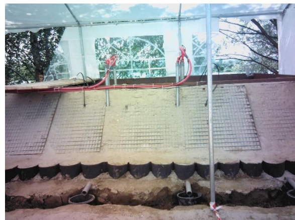
Fig. 4. View of the experimental embankment in visible spectrum.
