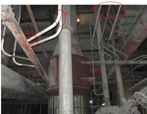
Fig.2. Example survey sites for inspection.
