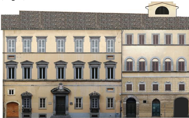
Fig. 2. The facade on via San Martino.
