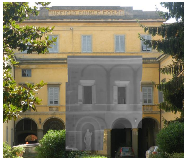
Fig. 6. Superposition of IR and visible images of the facade fronting the Arno river.
