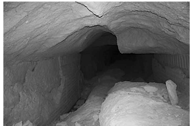
Figure 8. Fall from the vault, occurred at the intersection between two discontinuities.
