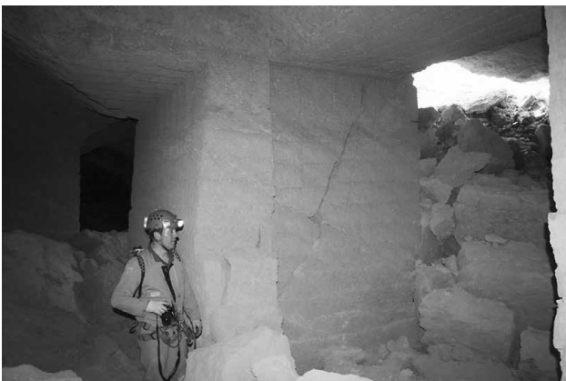
Figure 7. Cracks crossing a pillar; along primary (clinostratification, dipping to the right in the picture) and secondary (open cracks) discontinuities.
