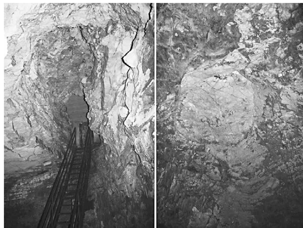
Figure 2. Examples of detachments from the vault of natural caves.
