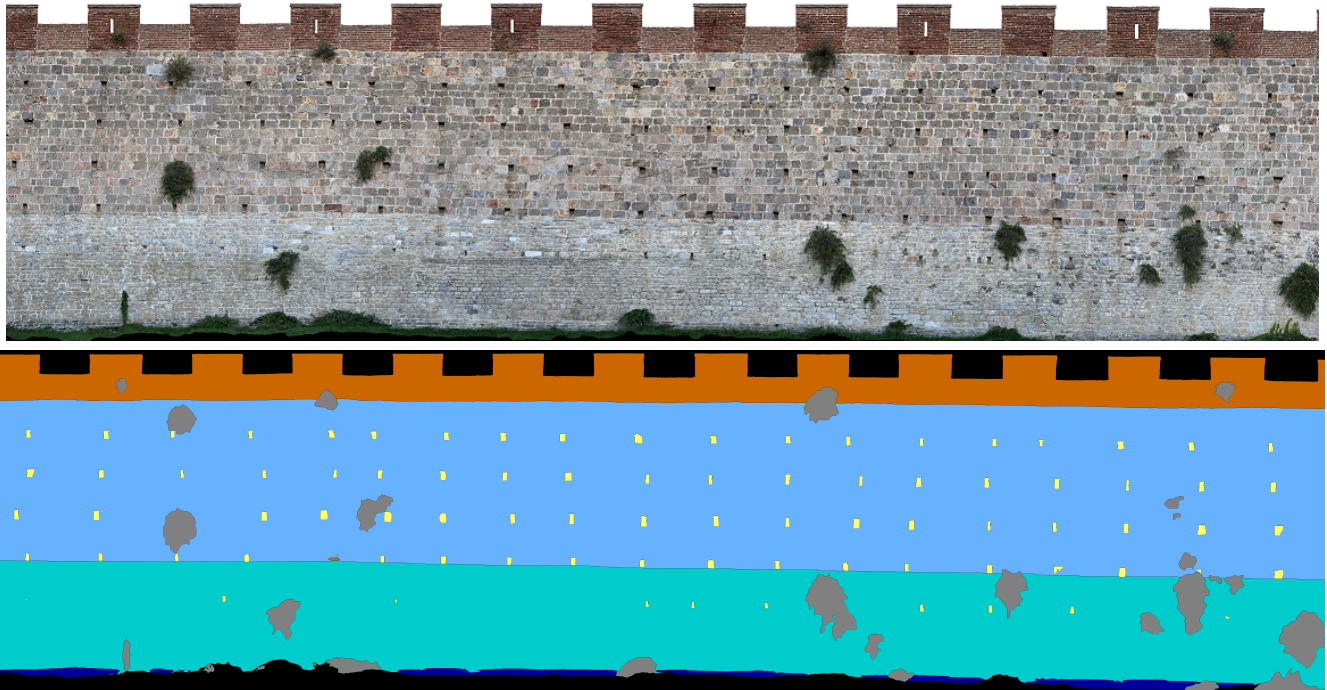
Figure 8: The Vittorio Veneto F ortho-image and the automatic masonry predictions map exported from TagLab as an image.
