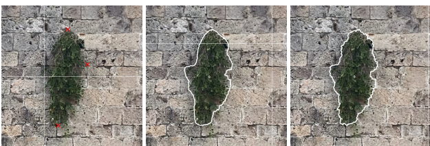
Figure 3: The 4-clicks segmentation tool in action. (Left) The user marks the extremes points of the area to be segmented. (Middle) The Deep Extreme Cut CNN automatically traces the boundaries. (Right) The Refinement tool can then be used to obtain a more precise segmentation.
