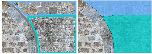
Figure 4: The Watershed tool in action. The azure and cyan scribbles mark two areas belonging to specific classes, while the grey scribble marks a "background" area to be ignored. The watershed algorithm transforms the scribbles into segmented areas.
