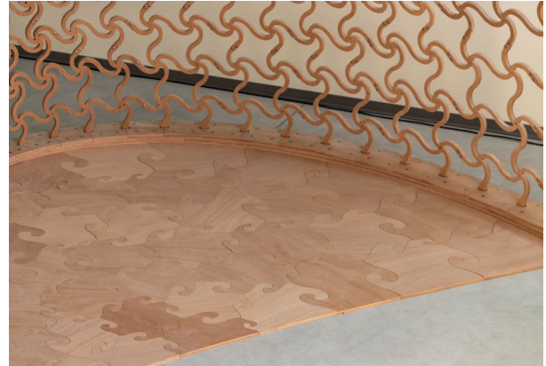
Figure 5: Variable-density interlocking Voronoi paving tiles.
