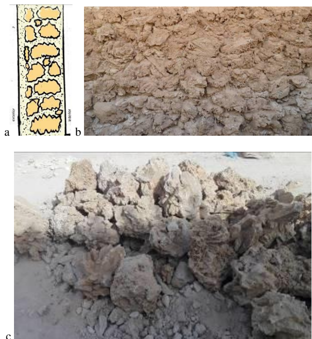
Figure 8. a. Section of 'Desert Rose' stone masonry. b. Wall of masonry building. c. Big 'Desert Rose' blocks.
