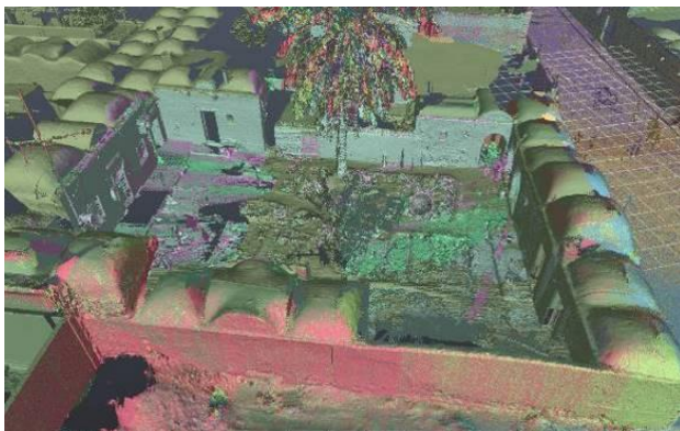
Figure 7. 3D survey of a typical minor building courtyard.
