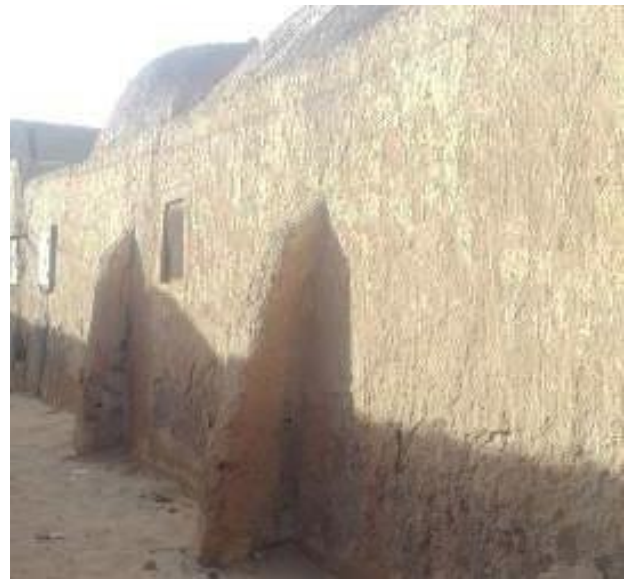
Figure 12. Buttresses of the wall overlooking the alleys.
