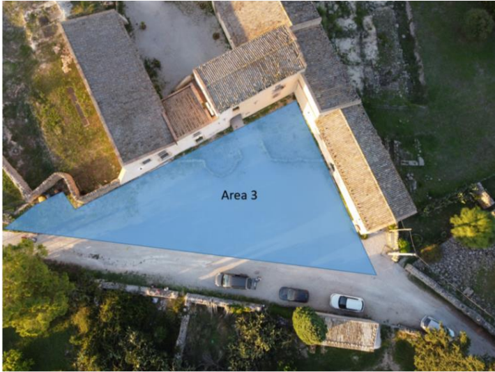
Figure 33. Aerial photo with indication of the limits of Area 3.
