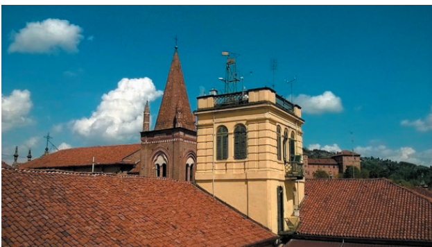
Figure 3. The tower of meteorological observatory in Moncalieri, managed by SMI (photo SMI, 11.04.2016).
