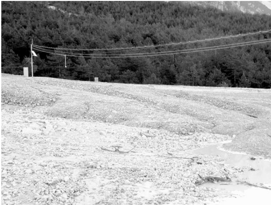
Figure 5. Downstream view of station 5; solar panel, data acquisition unit, steel cable and suspended ultrasonic sensor in foreground
