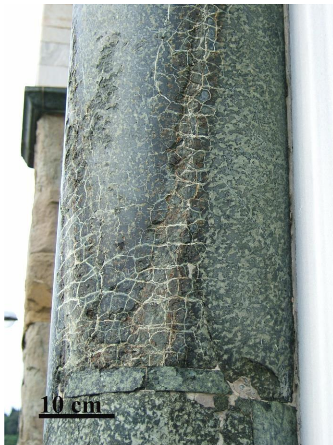
Figure 28. Veins of chrysotile which favour the detachment of fragments (Badia Fiorentina, Fiesole)
