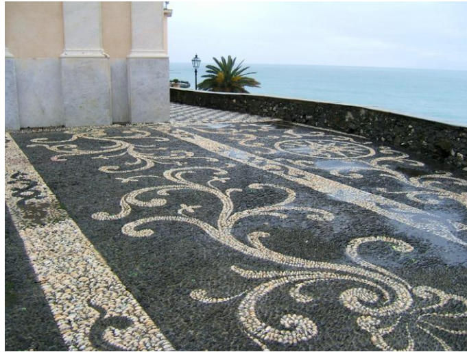
Figure 17. Bogliasco, churchyard of the parish church of Nativity with a "rissêu" decoration in white marble and green serpentinite pebbles dating back to 1767
