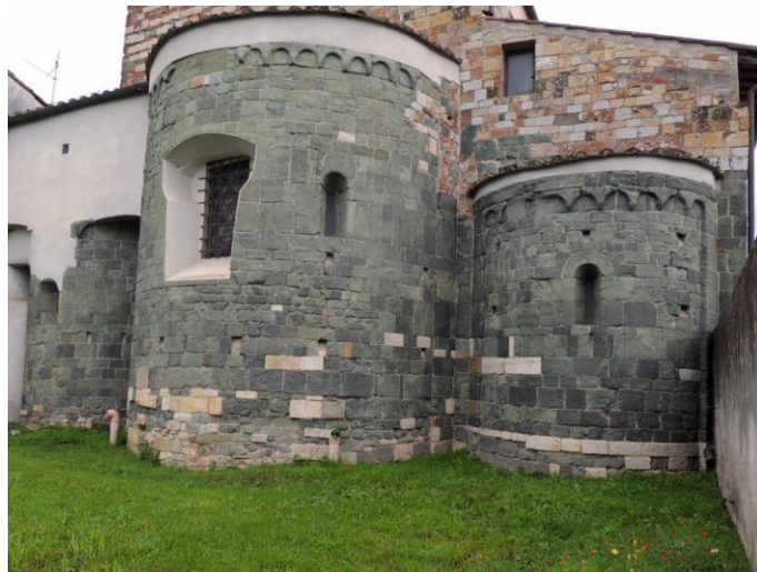
Figure 21. Church of Sant'Ippolito in Piazzanese where the serpentinite has been used as regular blocks in the masonry (Galciana- Prato) (XI century)
