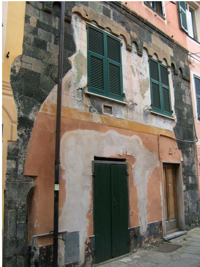
Figure 9. Merchant building of the XIII th -XIV th century where the serpentinite was used as regular blocks in the masonry (Levanto)
