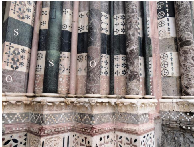
Figure 26. The gothic portals of the façade of San Lorenzo Cathedral in Genoa (XIII century) (where: S = serpentinite; O = ophicalcite)
