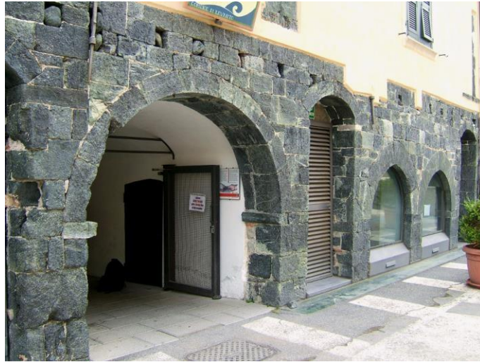
Figure 12. Levanto, former convent of the Augustinians, where the serpentinite was used as regular blocks in the masonry
