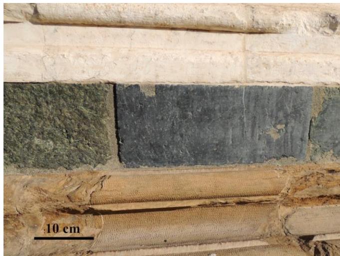
Figure 31. Substitution of a serpentinite ashlar with an Alpine serpentinite (Church of Santa Maria Novella, Florence)
