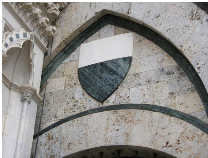
Figure 22. The Gothic portals of the Palazzo Pubblico with the "Balzana", emblem of Siena, where the dark half is made of serpentinite
