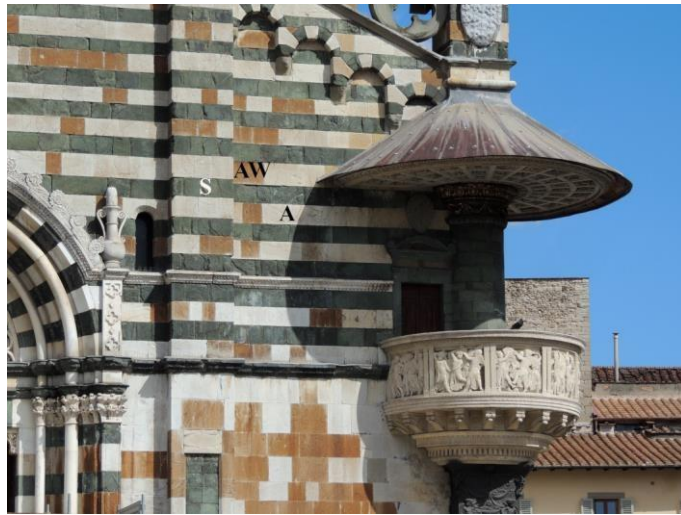
Figure 20. Prato, the bichrome cladding of the Cathedral of Santo Stefano with the Donatello and Michelozzo pulpit dating back to the first half of the XV century (where: S = serpentinite; A = Alberese limestone; AW = wheatered Alberese limestone)
