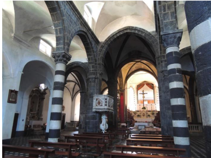
Figure 11. Levanto, interior of the church of Sant'Andrea, characterized by the use of serpentinite in the two massive pillars that delimit the presbytery and in the ribs of the vault, in the arches of the central nave, in the capitals and the dark strip of the columns
