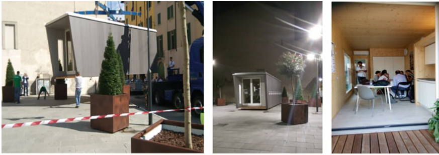
Fig. 3.6 Marlegno housing unit Nidoom installed into the city centre of Brescia during the ISS summer school, external view and internal view
