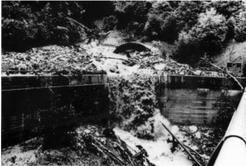
Figure 9. Debris flows often affect highways and motorways producing high risk situations as in the case of this Italian motorway severely damaged by a debris flow occurred on June 1996 after an analogous event already occurred in 1990. Seismic detectors might be employed in this and similar cases as warning systems until structural and more definitive.
