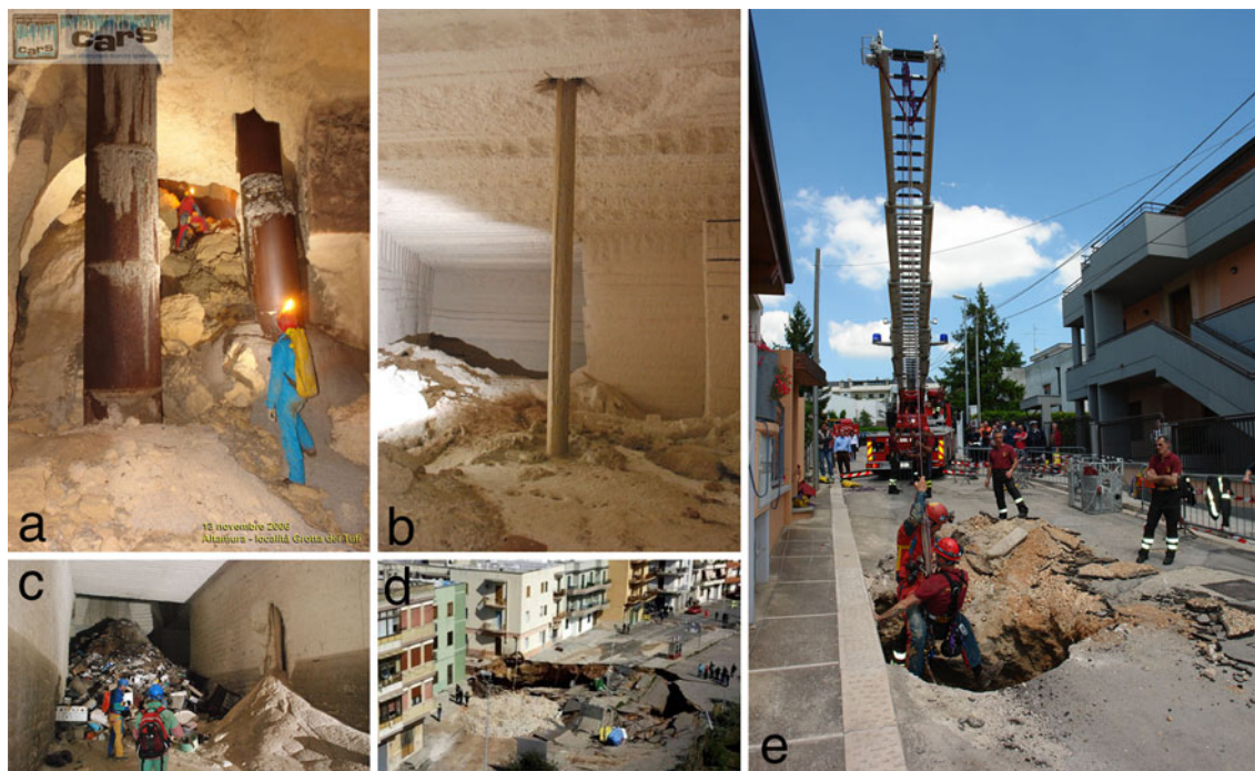
Fig. 3 Infrastructure at risk because of the occurrence of sinkholes related to underground quarries: a and b foundation piles within underground quarry at Altamura (photo courtesy of CARS) and Cutrofiano; c solid wastes in underground quarry at Cutrofiano;
