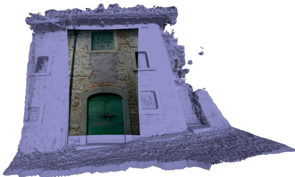
Figure 12. Structure from Motion model from the photogrammetry survey of a case study building in the historic centre of Cornillo Nuovo—SISMI project [41].
