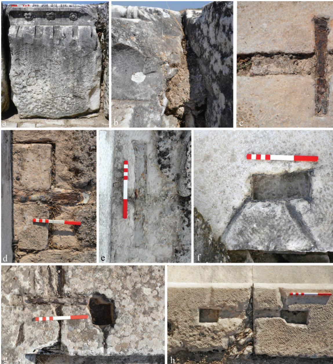
Fig. 13 Hierapolis, Temple A, bedding mortar used to fill the space between the orthostates (a. b) and the socle blocks (c); metal clamps not covered by the cella socle (d. e); two contiguous dowel recesses (f); dowel recesses close to the already placed clamps (g. h)
