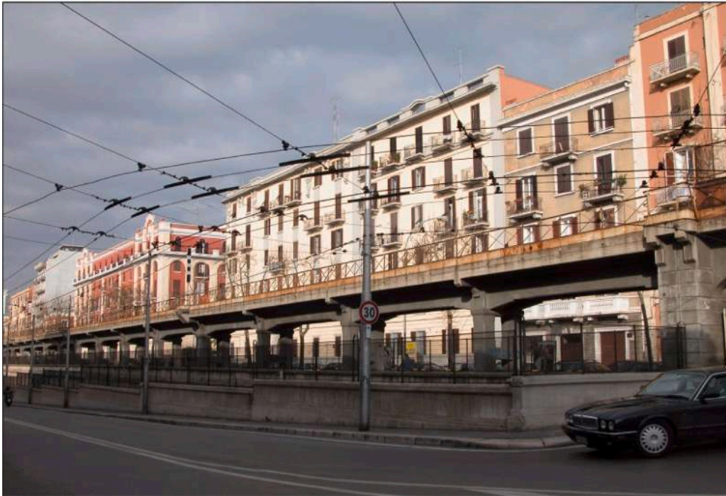
Fig. 2. An example of historical RC bridge made with Hennebique technique: Viaduct of Corso Italia, Bari, Italy.
