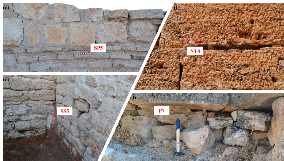
Figure 4. Some examples of (a) bedding mortar (SP5 sample—Church of St. Philip); (b) grouting mortar (NT4 sample—Nymphaeum of the Tritons); (c) coating mortar (SS5—Stoa of the Springs); and (d) concrete fill (P7 sample—Ploutonion).
